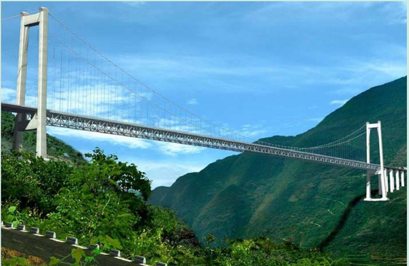
Fig.1: General view of the Balinghe Bridge. • Photo: Tongji University
